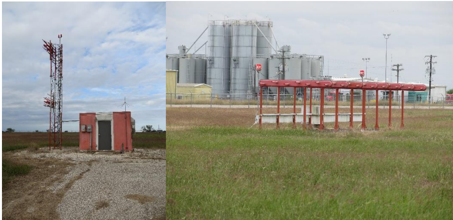
Victoria Regional Airport Glideslope Antenna (left) and Localizer (right).
